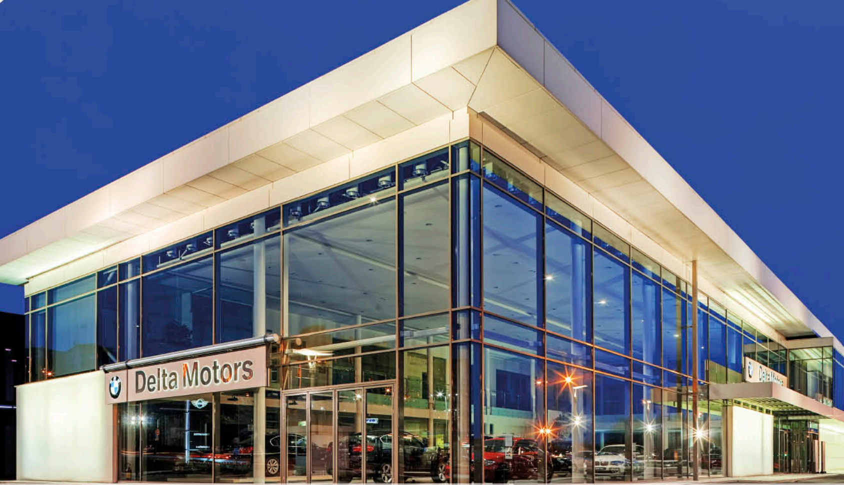
Godina izgradnje / Year of build: 2008 Investitor / Investor: DELTA Motors Arhitekta / Architect: Mašinoprojekt Kopriv, Beograd Fasada / Facade: 1.300 m 2 Krov / Roof: 3.700 m 2
