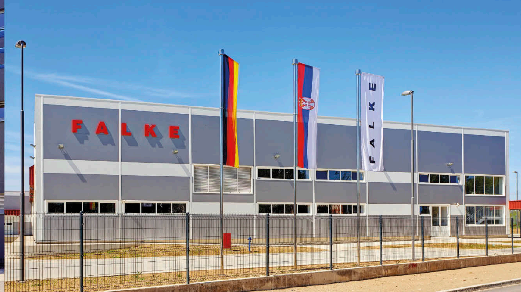
Godina izgradnje / Year of build: 2011 Investitor / Investor: Falke Serbia Projektovao / Design: Mašinoprojekt Koprings, Beograd Fasada / Facade: 5.500 m 2 Krov / Roof: 13.000 m 2
